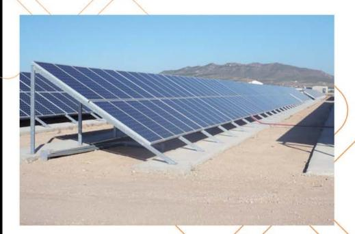
The Enersol's ballasted structure is the best solution for the execution of the foundations in slightly cohesive terrain, due to the low connection between its particles, it is necessary a bigger support that distributes the loads.
