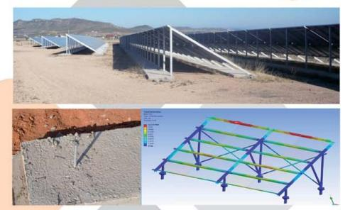
In the foundation a threaded bar is placed in the concrete like a start rebar; in which the structure of the photovoltaic modules is assembled, by means of a "multipoint system", which allows to regulate enevenness and differences in three directions (x, y, z).
